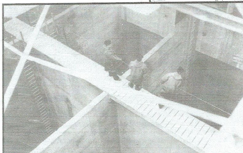
Partitioned sections of the 'Pheonix' caissons internally to a depth of 50ft/15.2 mtrs. When in position off Arromanches the sea valves were opened, sinking them on the seabed.
