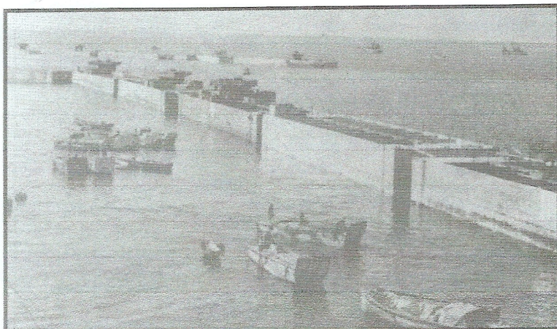
The inside of the harbour protected by the sunken 'Phoenix' caissons. In the background is the outer wall of the sunken caissons forming an entrance to the harbour.
