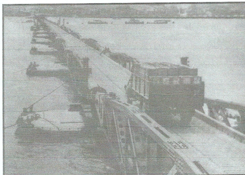
This photo shows the floating pontoons with the steel bridges joined to each pontoon. These bridges were designed so that in rough weather they could move up and down with the wave motion.
