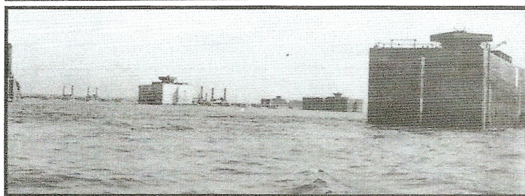
5th June 1944 'Phoenix' caissons and 'Spud' pontoon pierhead in the background off Pagham ready to leave next day for Arromanches.
